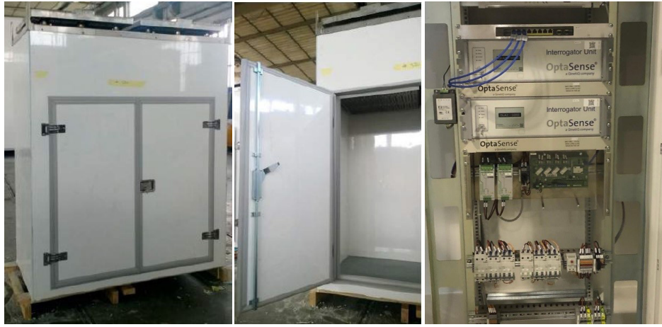
Installation of the OptaSense pipeline monitoring equipment inside a passive cooling cabinet.
